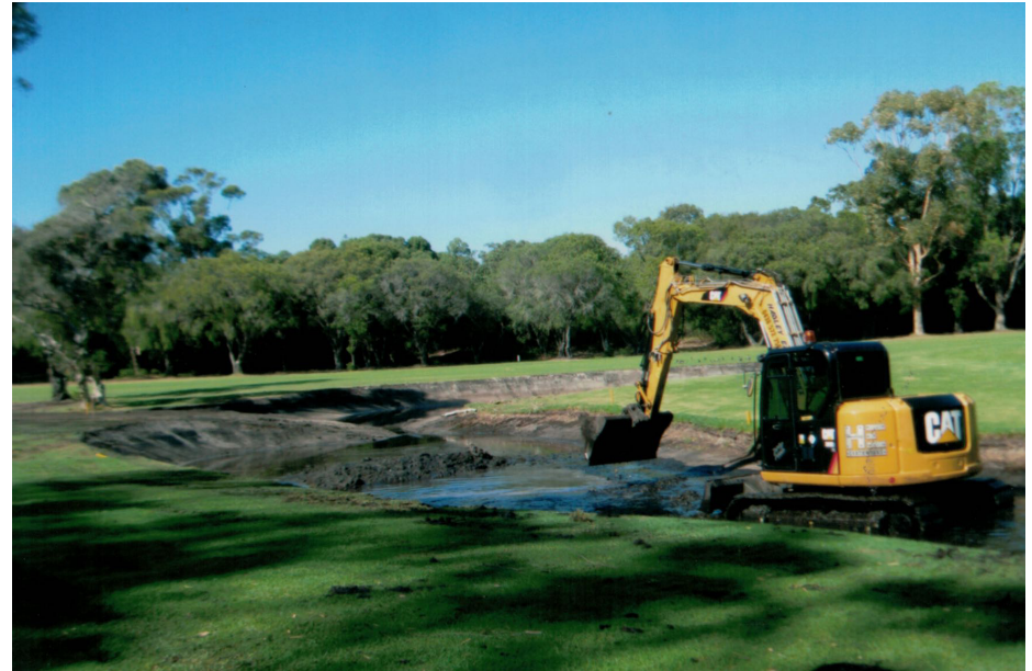
March 2017 - Enlarging the lake at the front of 8 green.
