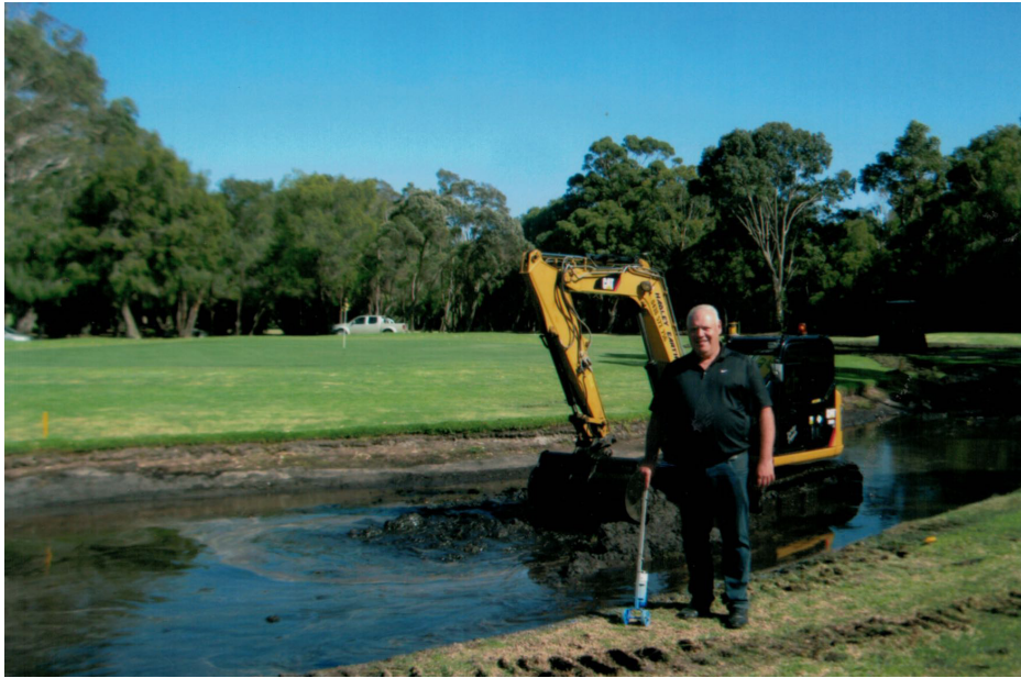
March 2017 - Earthworks done to establish new lakes along 7 and 9 fairways
