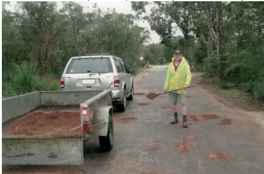
2016 - Ray repairing original road by filling in potholes with gravel.
