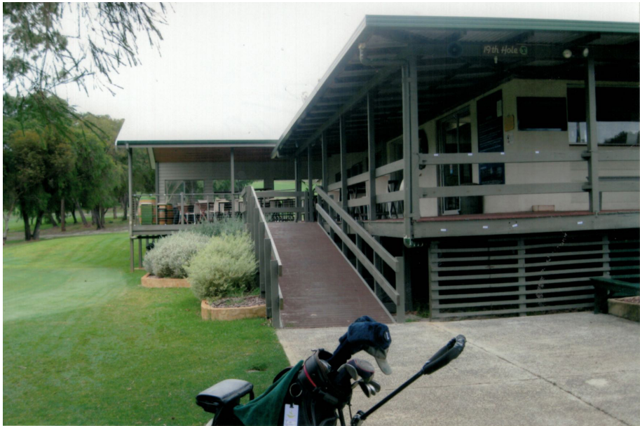
2012 - New Ramp put onto the extension, stairs taken out.
