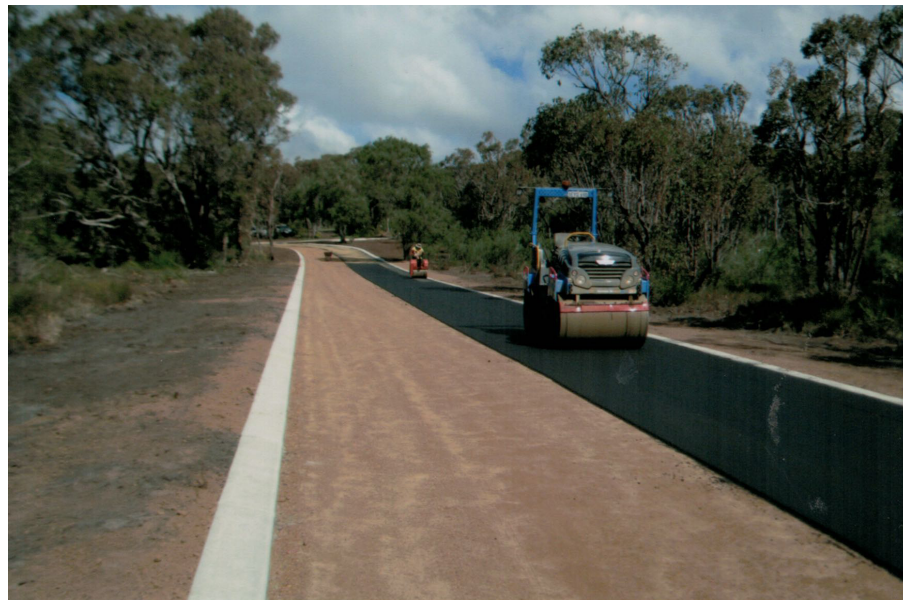
2018 - The new road put in as part of the NBN Tower deal. Compare to machinery used 33 years earlier
