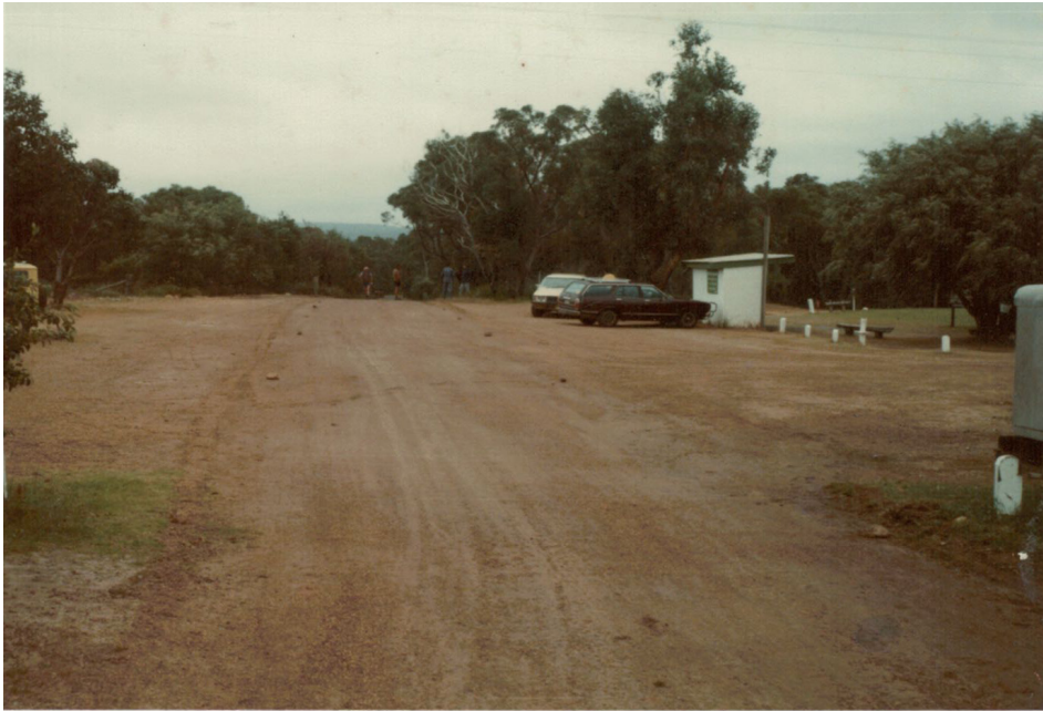
1985 Preparing the original golf club road to be bituminised.
