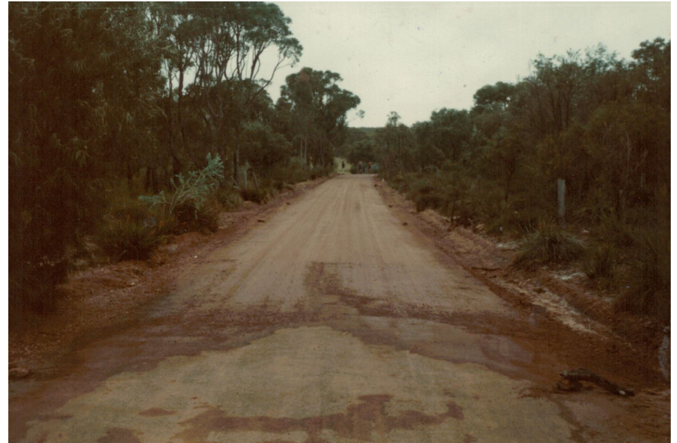
1985 The road entrance before sealing.
