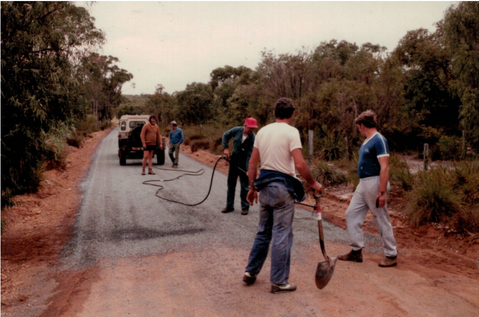
1985 Putting out the blue metal at the entrance
