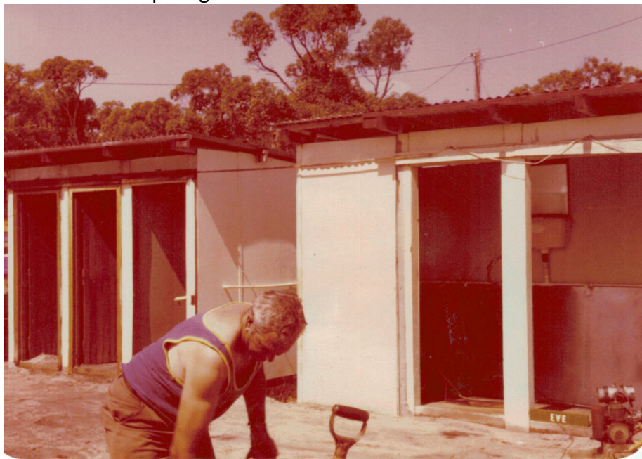
1979 Clubhouse new toilet block being built, Doug Phillip-Jones mixing cement
