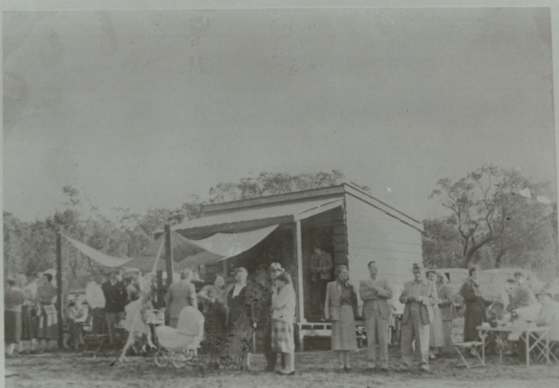
The original clubhouse 1955
